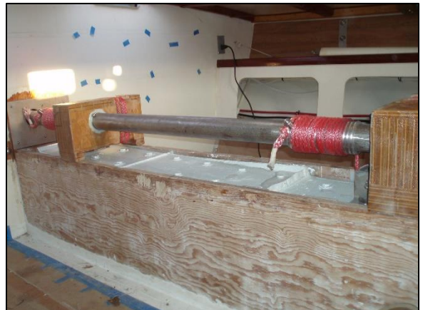
Support beams on trunk ( under constr'n. ) ←
